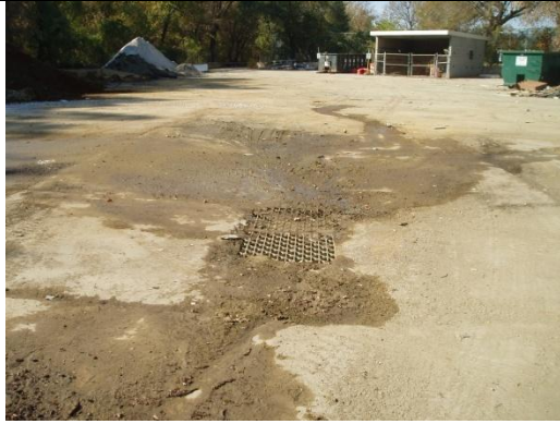
Unprotected storm drain inlet
