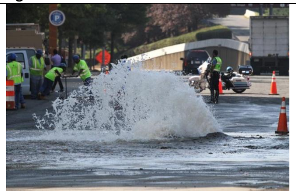
Figure 10. Water main break
