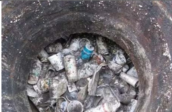
High Severity Waste Management – Trash clogging storm drain manhole.
