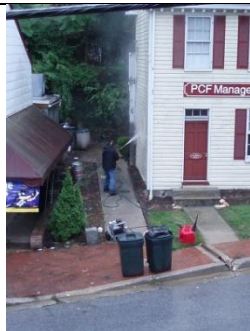
Low Severity Washing – Individual power washing building side without soap
