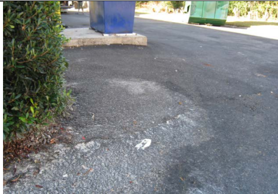
High Severity Waste Management – Grease accumulation on lot draining to storm drain
