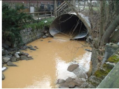
Severe Severity Sediment Discharge
