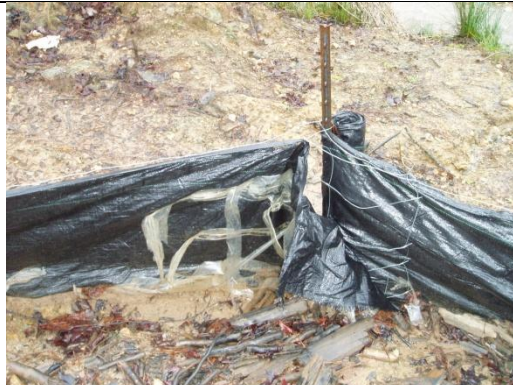
Failing silt fence
