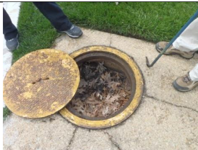
Moderate Severity Yard Waste Management – Clogged storm drain
